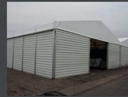
Flexistrukture – external building
