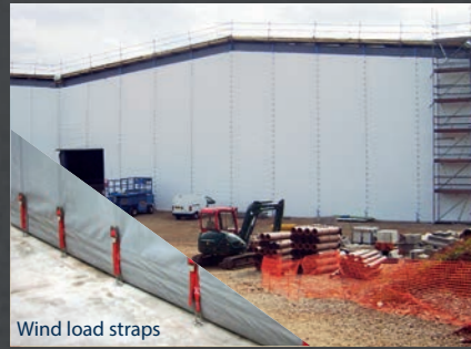
Flexiscreen – internal or external temporary building dust screen
