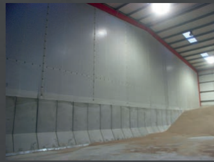
Flexiwall – above rocket wall for dust control
