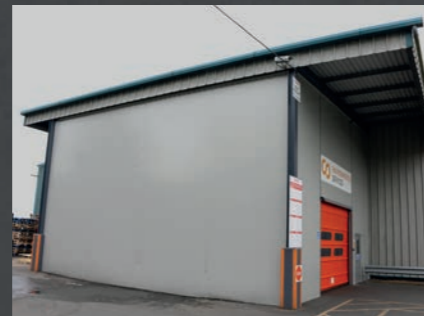
Flexiwall – external canopy enclosure
