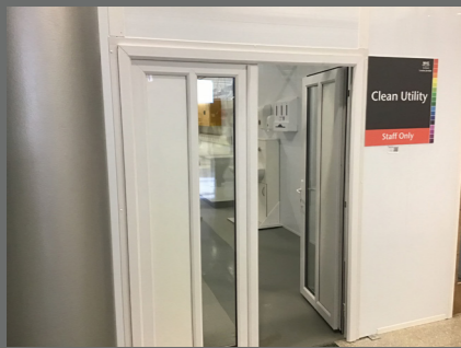
Fire rated hoarding to comply with fire regulations
