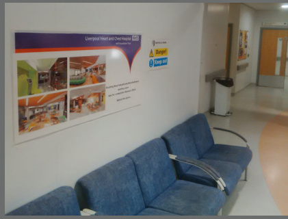
Acoustic hoarding for sound reduction in public areas
