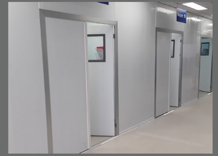
Floor-to-ceiling hoarding for infection control
