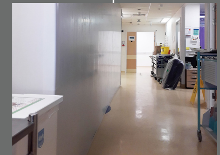
uPVC floor-to-ceiling hoarding for dust control during refurbishments
