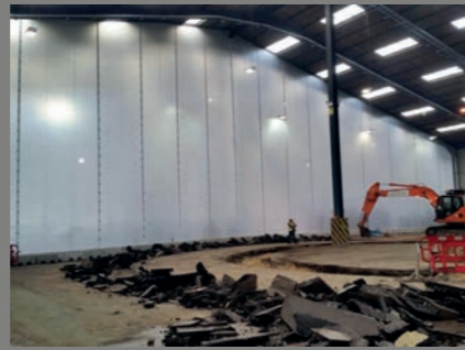
Flexiscreen – temporary screen for building works (internal and external)
