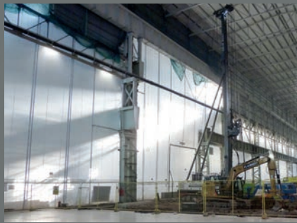
Flexiscreen – temporary screen for building works (from the inside)
