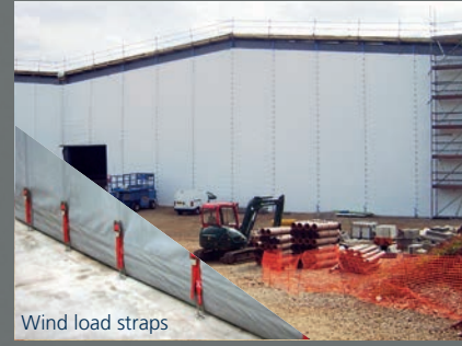
Flexiscreen – temporary screen for building works (from the outside) Wind load straps
